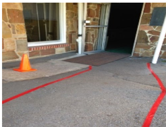
Duct tape designates access aisle as temporary measure. Photo courtesy of Disability Rights Texas.
