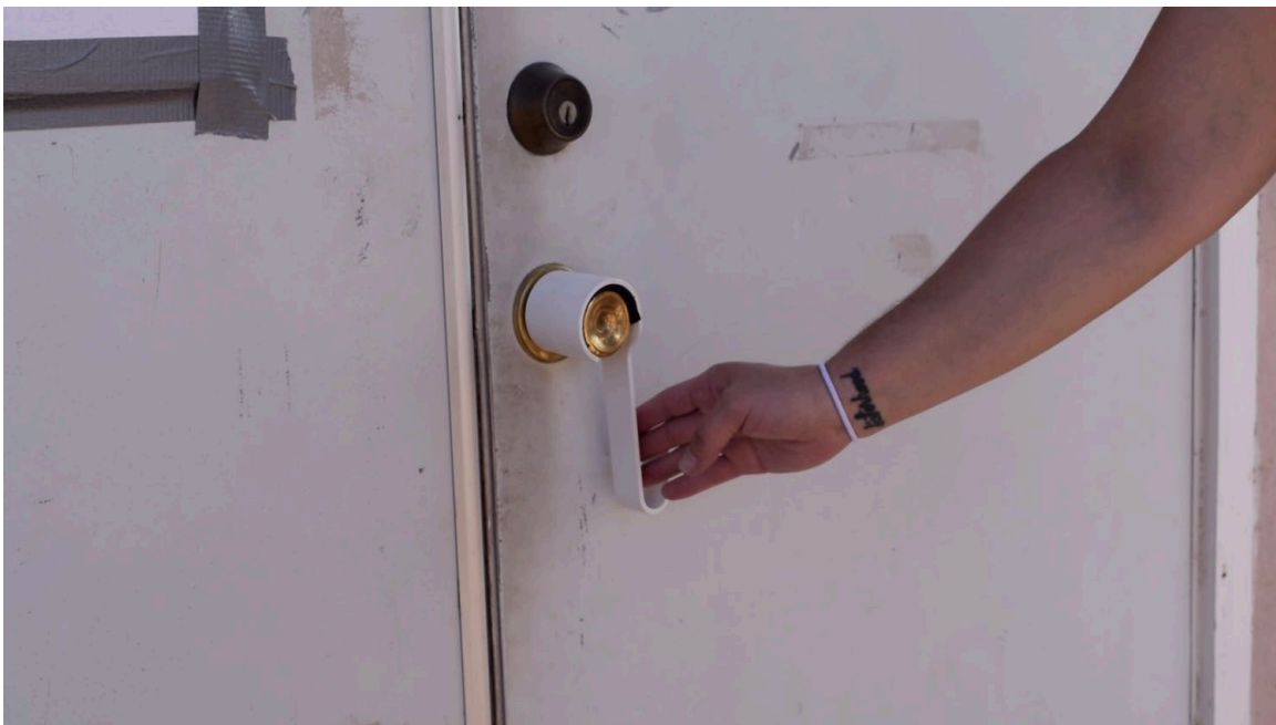
Round doorknob is outfitted with a retrofitted lever knob.
