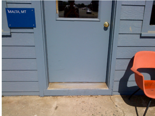
Photo 23: This step makes the entrance to the Malta Station inaccessible.
