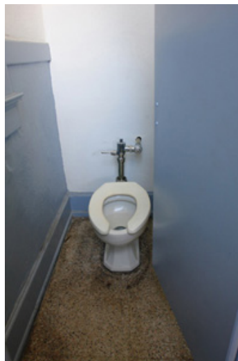
Photo 5: Inaccessible restroom in Tuscaloosa station.
