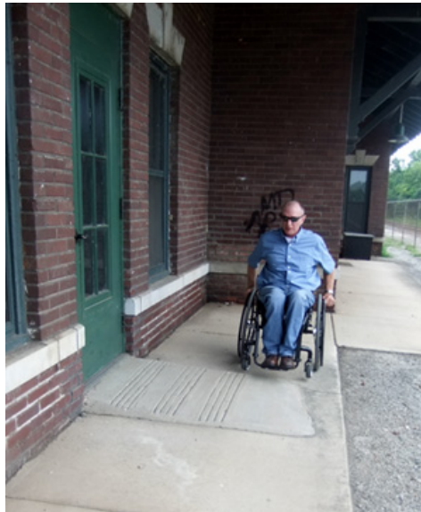
Photo 6: Ramp crossing into path of travel at Arkadelphia station.
