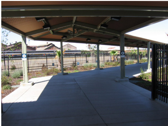
Photo 10: Travel path to platform (continued).
