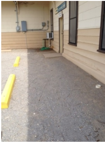
Photo 37: Irregular brick platform at McGregor station.
