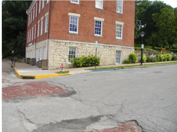
Photo 20: The accessible parking space at the Jefferson City station is located on a slope rather than a flat surface.
