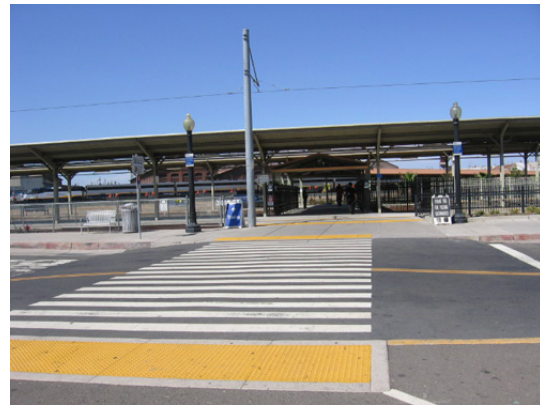
Photo 9: Travel path to platform (continued).
