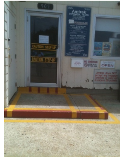
Photo 35: Inaccessible entrance to the Longview station.
