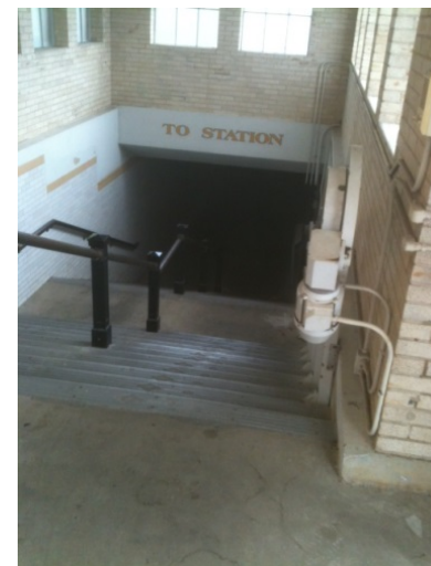
Photo 36: Stairs are the only access to the Marshall station.
