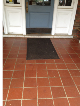
Photo 41: This step at the Ashland station makes the entrance inaccessible.
