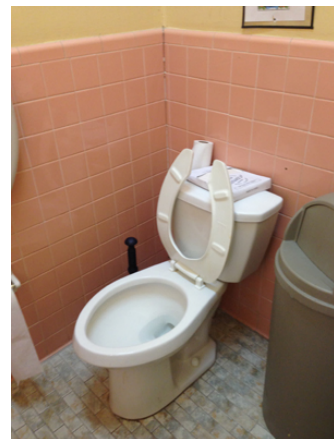
Photo 15: No grab bars in restroom at Kissimmee.
