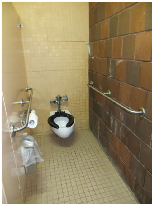
Photo 32: The restroom at the Cleveland station seen in this photograph is not accessible.
