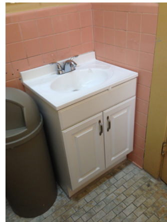
Photo 14: No clearance to access sink at Kissimmee.
