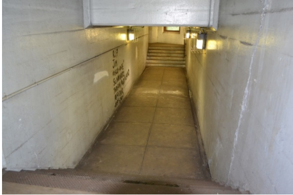
Photo 3: This tunnel is the only access between platforms at Harpers Ferry station.
