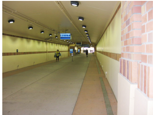
Photo 11: Travel path to platform (continued).
