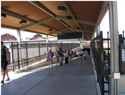
Photo 8: Travel path to platform
