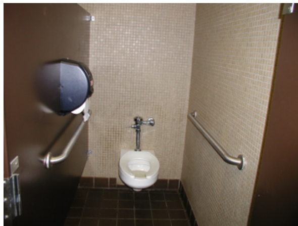
Photo 21: This restroom stall at Jefferson City station is too narrow for a wheelchair.
