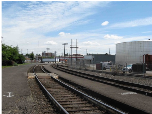
Photo 43: Deteriorating pavement at the Vancouver station.
