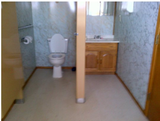
Photo 24: Narrow restroom stall and inaccessible sink.
