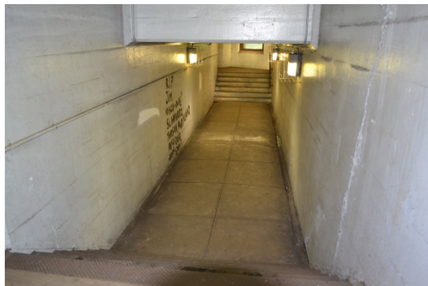
Photo 46: This tunnel is the only way to get from one side of the tracks to the other at Harpers Ferry station.
