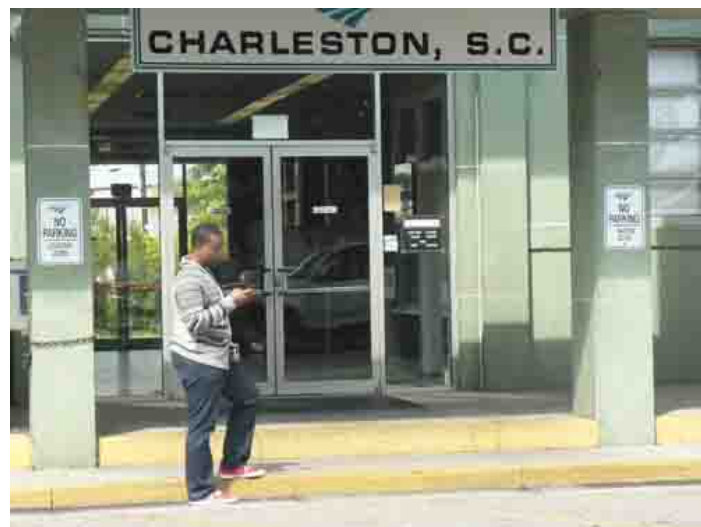
Photo 34: Steps at the entrance of Charleston station make it inaccessible.
