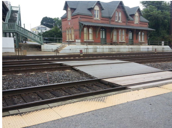
Photo 12: A stairway and bridge on left are the only way to get from one side of the platform to the other.
