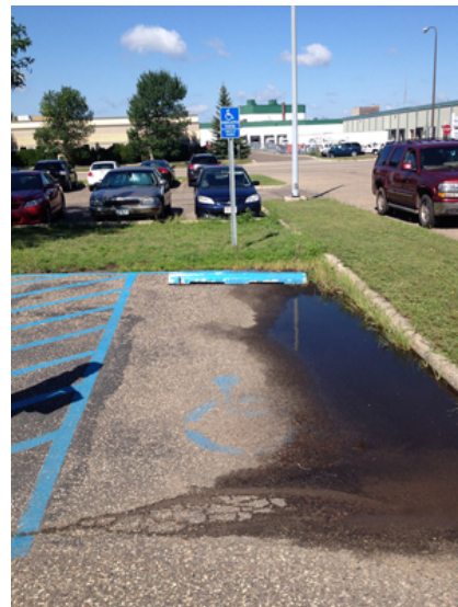
Photo 19: Unlevel parking space at St. Paul station.
