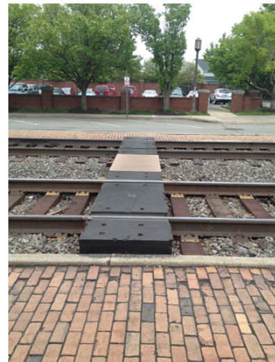
Photo 42: This walkway at the Ashland station is inaccessible to wheelchair users and others with mobility-related disabilities.
