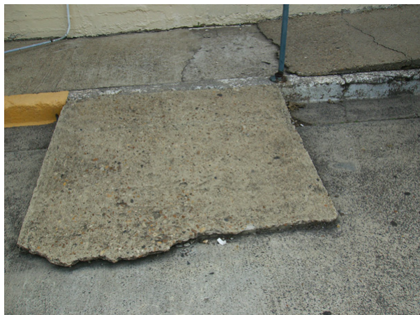
Photo 7: Crumbling ramp at Texarkana station.
