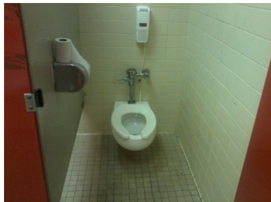
Photo 30: Restroom stall at the Rochester station is too narrow for a wheelchair user, lacks grab bars and has a toilet paper holder mounted too high.
