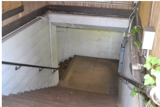
Photo 47: Stairs to platform at Harpers Ferry station.
